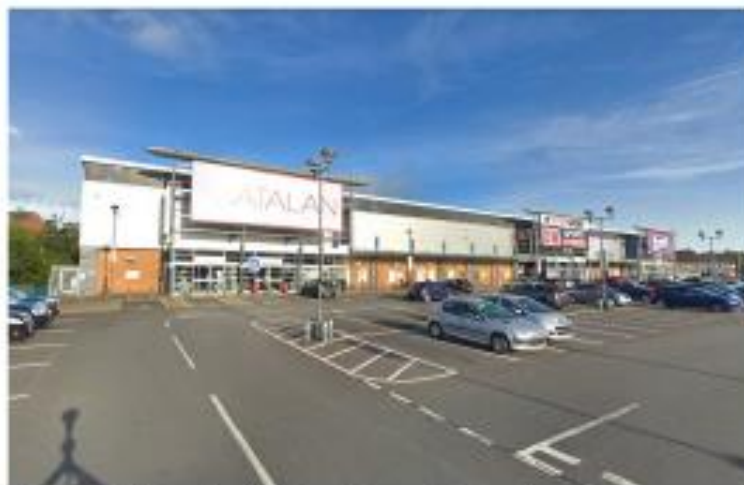
Photograph | View of retail units off Caernarfon Road
