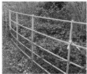
Precedent for new low level fencing type (boundary to new car park)
