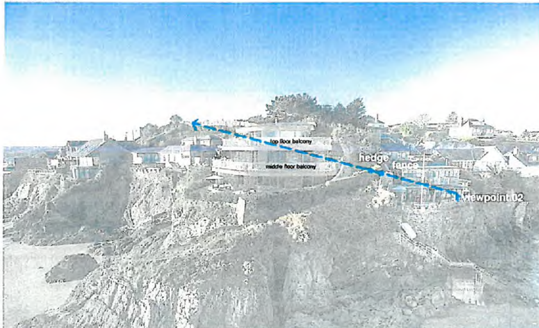
view from north east
